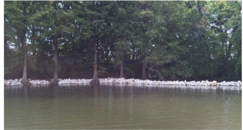
LAKE SPRINGFIELD SHORELINE STABILIZATION USING ROCK RIP RAP
